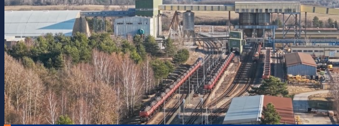
Rail loading yard at the smelter
